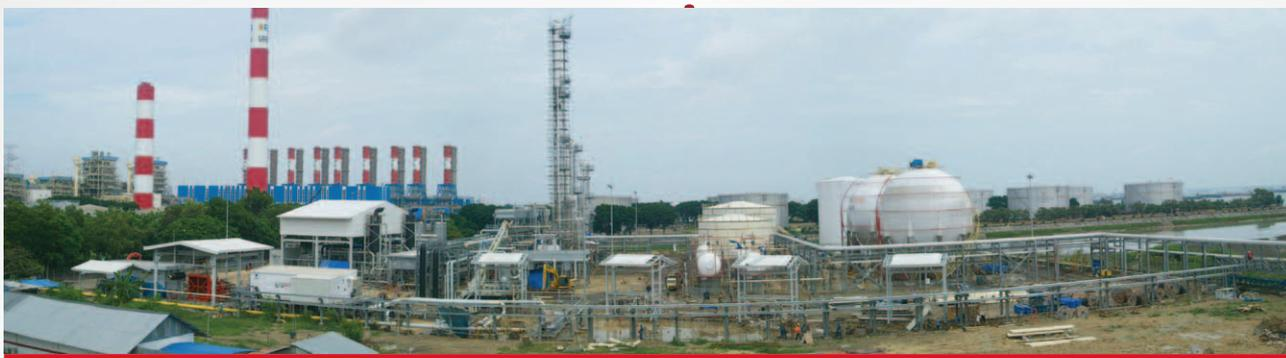
This cryogenic plant in Surabaya, Indonesia, was designed by Valerus to withstand seismic activity while extracting hydrocarbon liquids.
